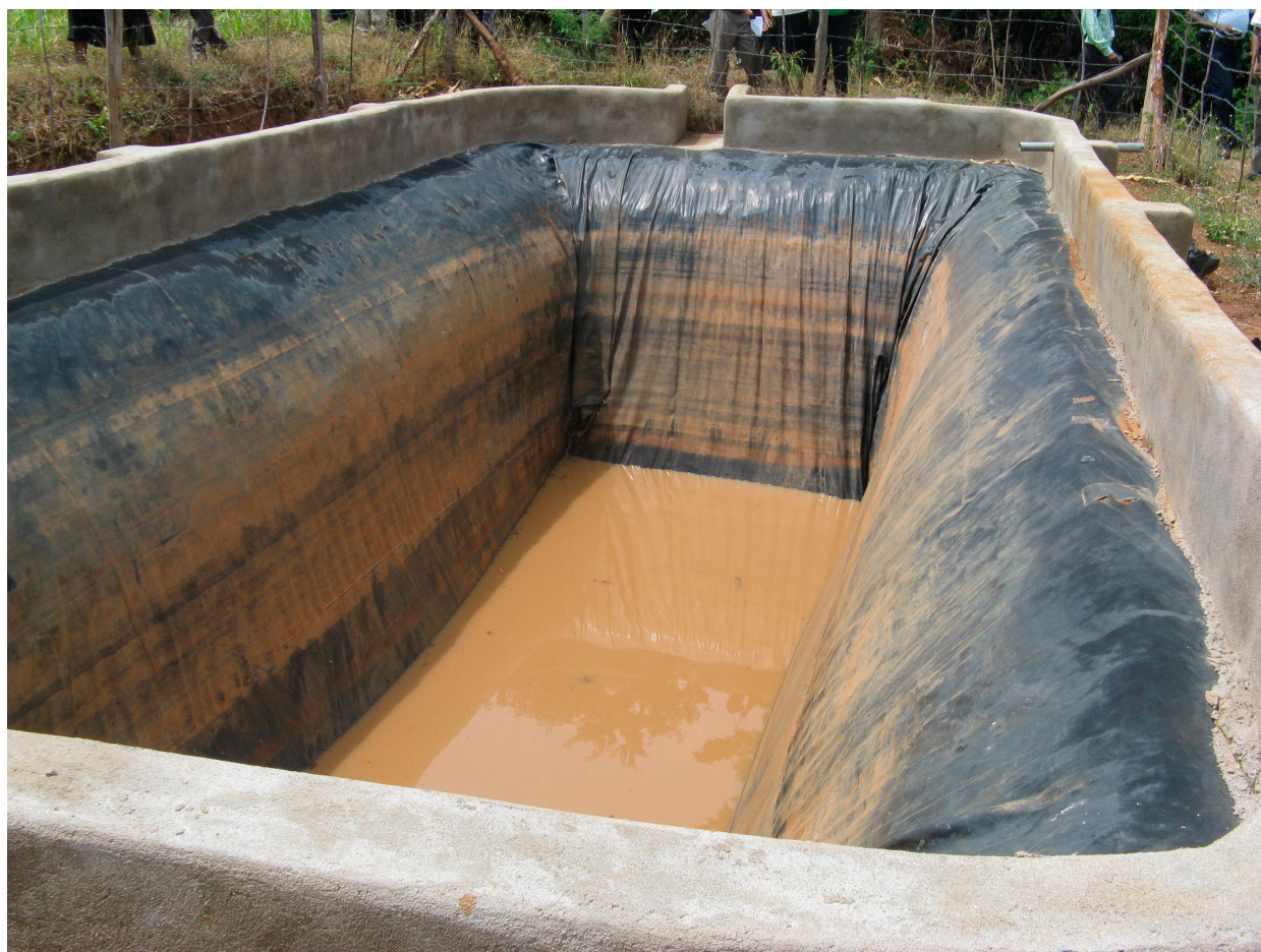
Figure 13. Plastic-lined pond for rainwater collection used in harvesting surface runoff for irrigation in Tanzania. Ponds should be covered to (i) minimize evaporation loss, (ii) protect harvested water from vagabonding animals, and (iii) avoid drowning of children. Own archive photograph, taken in Kilimanjaro region.
