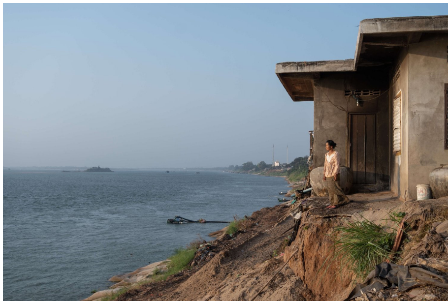
Abb. 2: "Hak Bopha, a grocery and gravel seller, stands for a portrait behind her house, which was partly destroyed by a riverbank collapse on the banks of the Mekong river. A few hundred metres away, dozens of barges pump sand at Rokar Koang Commune, one of the most heavily mined sections of the river in Cambodia" (Ball o.J.). © Andy Ball/University of Southampton.
