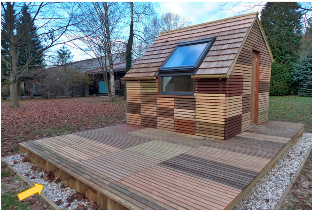
Figure 1. Wooden model house unit in October 2013 at the beginning of the exposure. Yellow arrow is pointing north.
