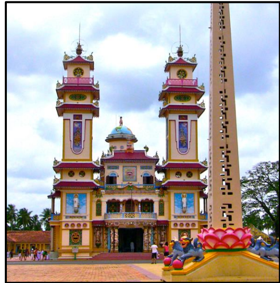
The Gothic façade at the entrance is a “European front” to an Asian interior.
