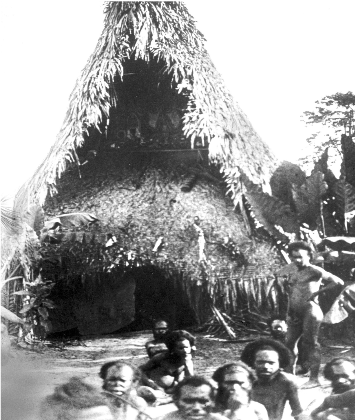
6. The Austrian-German ethnologist Richard Thurnwald passed through the Maprik region in 1913. He was the first to document ceremonial houses and their many variations. This ceremonial house in “Ambatigi” features a small gable painting and a pent roof covered by a plaited mat below the carved crossbeam. Photo: R. Thurnwald 1913.
