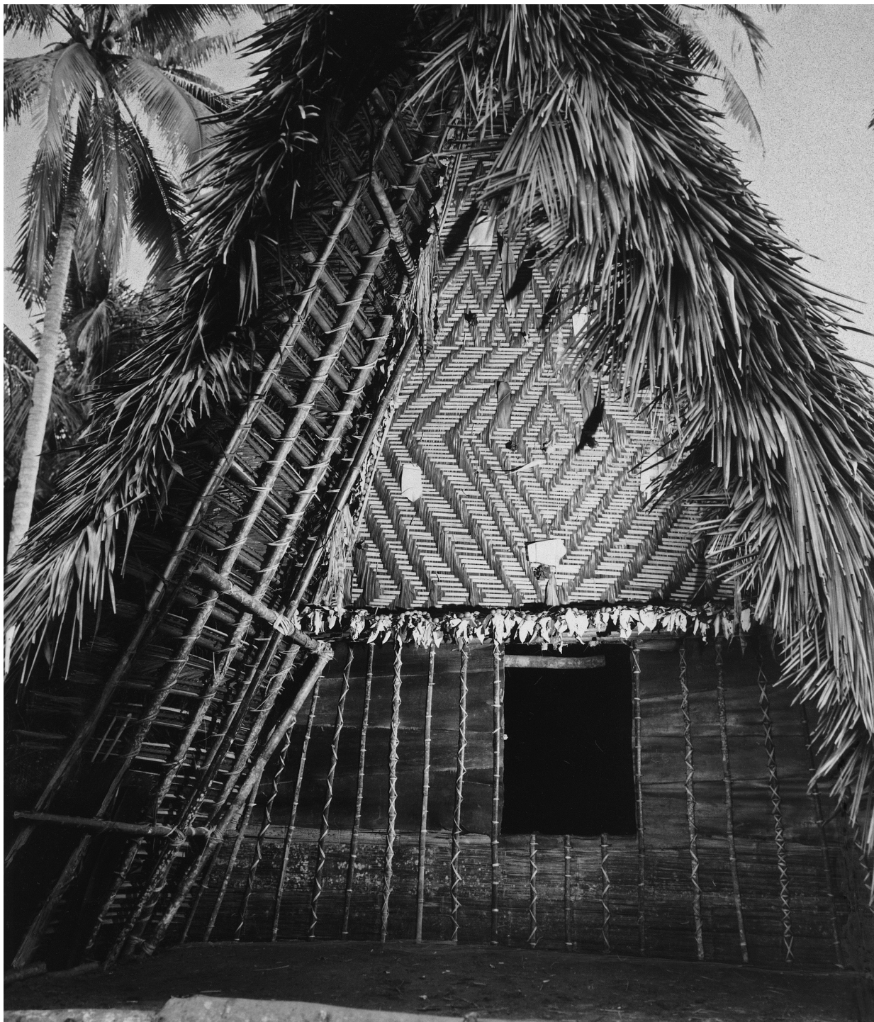
26. Storage house with plaited mat decorating the upper gable section. The lower part is covered by palm leaves sewn together with ornamental stitches.
